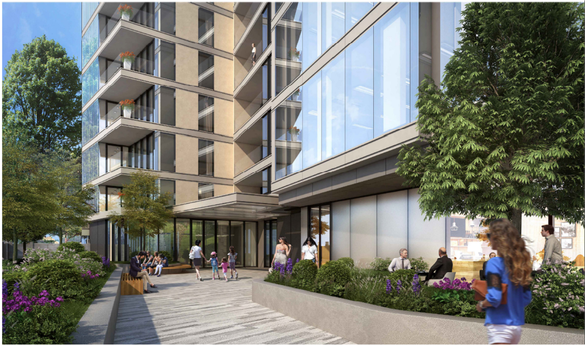
The access way to the residential flats
